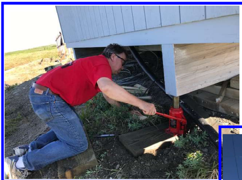
Leveling the Phasor Building at the Tower site
